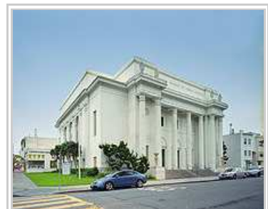
As of November 2009, new Internet Archive headquarters at 300 Funston in San Francisco, CA, a former Christian Science Church
