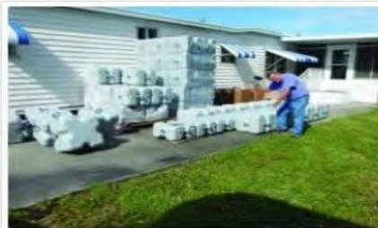
2. THE CENTER OF THE DOCK MUST BE ASSEMBLED ON A LEVEL, FLAT SURFACE. HALF BLOCKS IN THE CENTER ACCOMMODATE THE KEEL. THE OUTER FULL BLOCK ROWS ARE CONNECTED TO THE CENTER WITH PLASTIC BOLTS AND NUTS.
