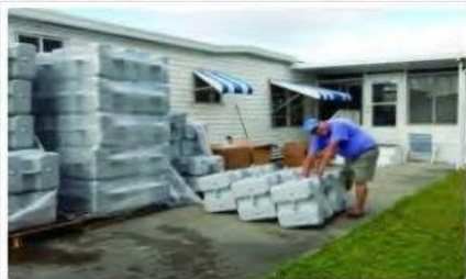
1. UNLOADING AND PREPARING BLOCKS. EACH BLOCK MUST HAVE A THREADED HOLE PLUGGED WITH A NYLON PLUG TO RENDER IT WATER TIGHT.
