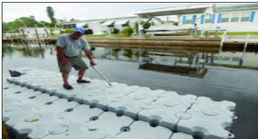
5. THE PINS THAT HOLD THE BLOCKS TOGETHER MUST BE TIGHTENED A QUARTER TURN TO LOCK THEM TOGETHER.
