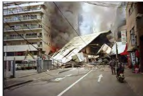
Burning and collapsed buildings in Kōbe, Japan, after the January 1995 earthquake. Dr. Roger Hutchison/NGDC
