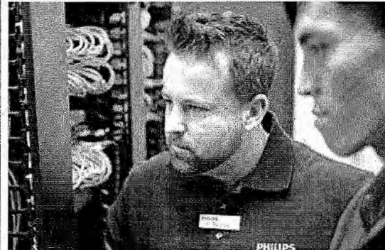
Bringing Value Added Services to the hospital server room
