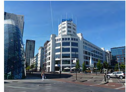
The Philips Light Tower in Eindhoven, originally a light bulb factory and later the company headquarters [19]
